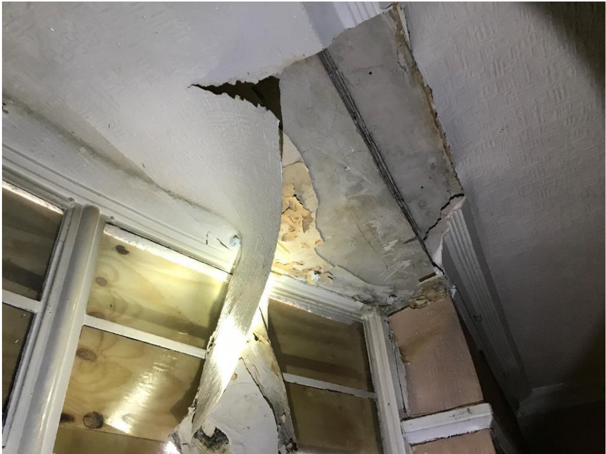
Roof leak / collapsing ceilings
